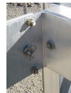
Stainless Pins with Grease Zerks
